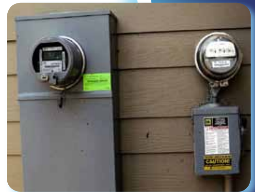
Figure 1: Typical location of Utility External Disconnect Switch, marked with a yellow caution label, below the production meter. The revenue meter is to left.
