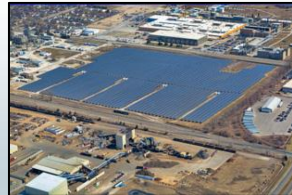
Maywood Solar Farm
