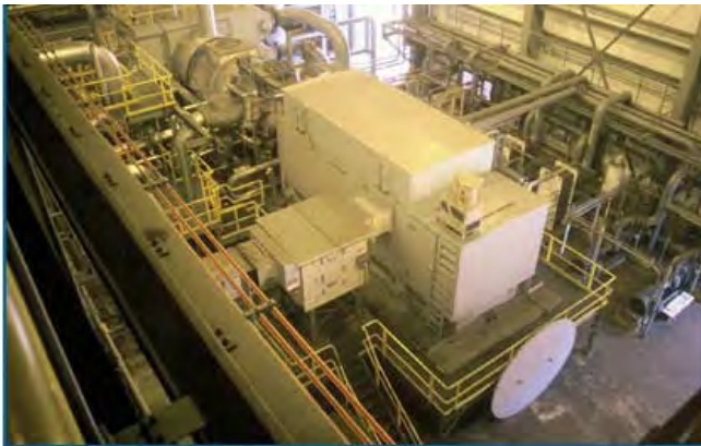
Cokenery's Installed WHP System at ArcelorMittal
