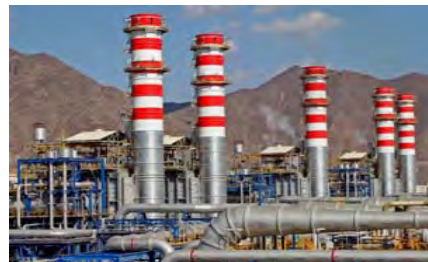
Natural Gas Power Plant 250 MW
