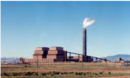
Coal Fired Power Plant 500 MW
