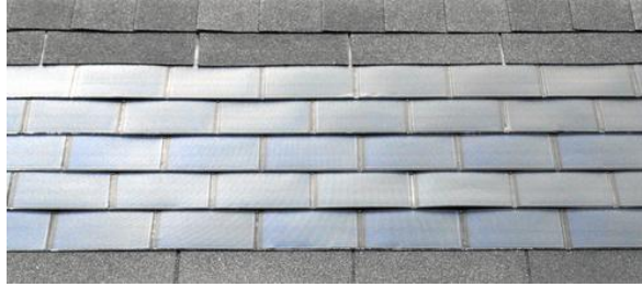
Figure 2. Thin-film solar PV shingles. Photo from United Solar Ovonic, NREL/PIX 13572
