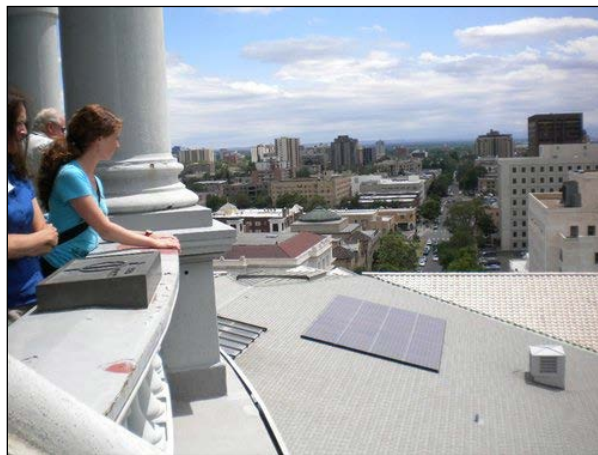
Figure 7. PV Panels on Denver Capitol Photo by Eliza Hotchkiss, NREL/PIX 18594
