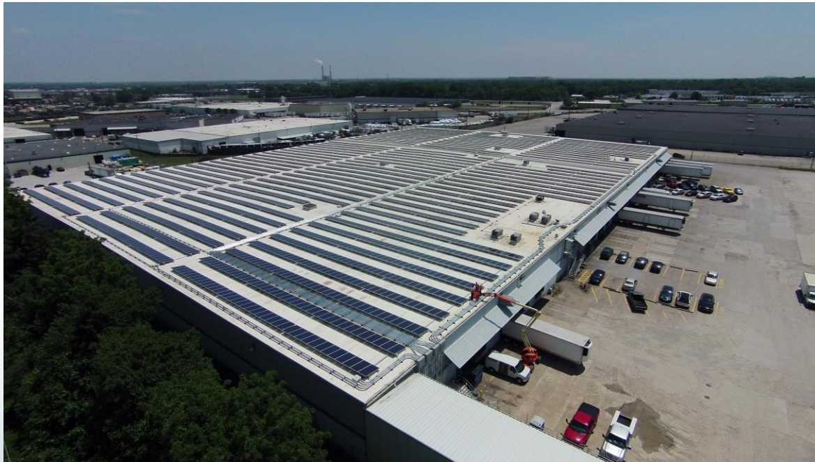
Grocers Supply Roof, 1MW rooftop system.
